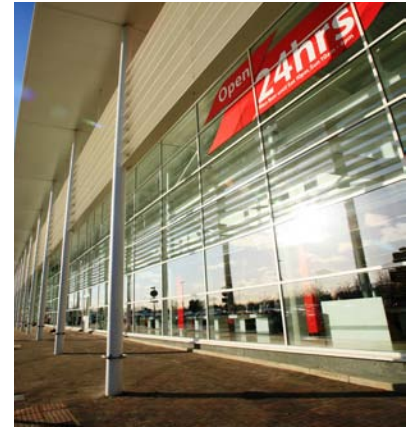
▲ Main Entrance Facade Glazing Terrace with Sollex HALO-vx1 Feature
